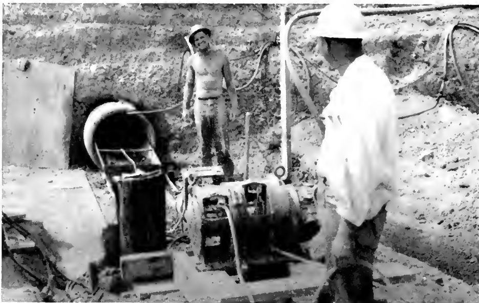
Sled and trigger winch used in removing excavated material
